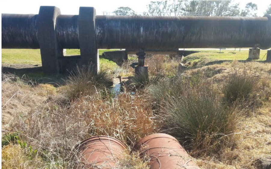
PLATE 4.3 - PIPE CROSSING AT WARRAGAMBA PIPELINE EASEMENT
